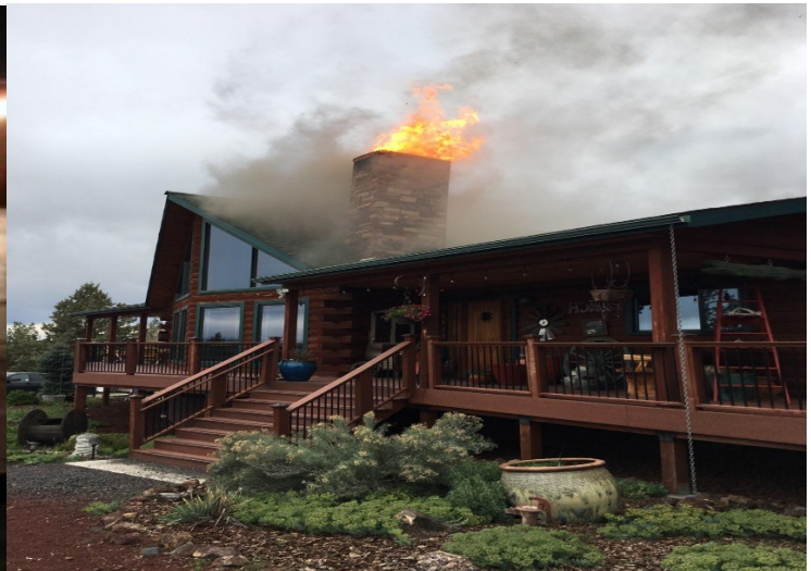
Chimney Fire on Dove Rd. this past May
